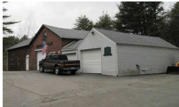
74 Warren Ave. The "Water Division Building"
