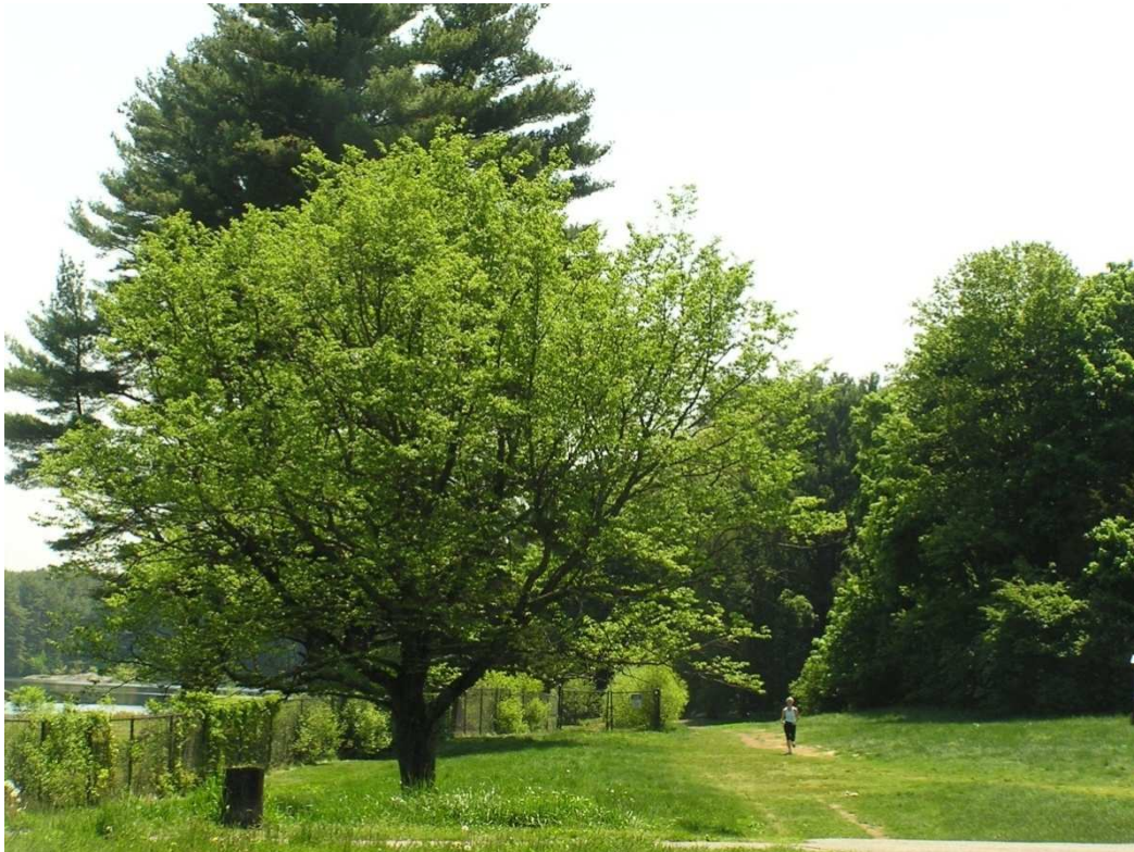
Trees on the earthen dam will be removed to prevent erosion
